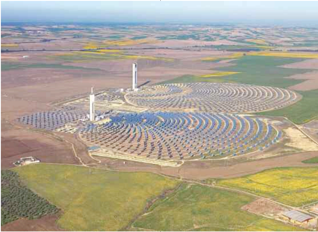
Solar energy towers in Seville, Spain.
