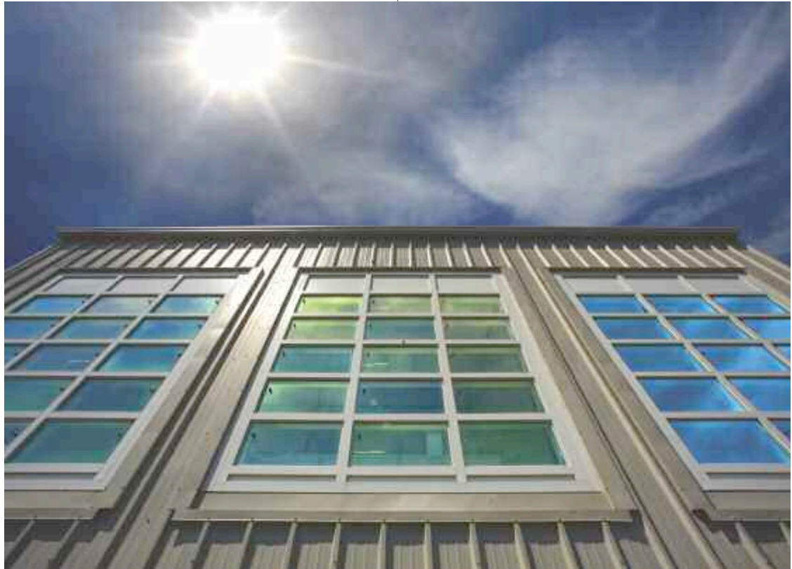
Energy-efficient windows at Lawrence Berkeley National Laboratory, California.
